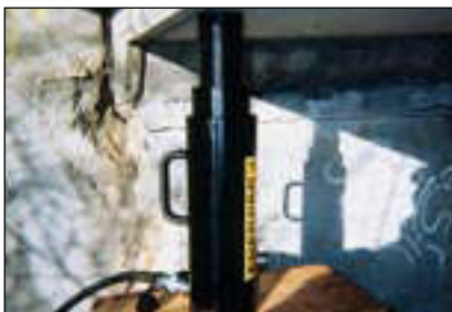
◀ The portable lock nut cylinder RACL-1506 used for extended load support during epoxy injection for bridge reinforcement.
